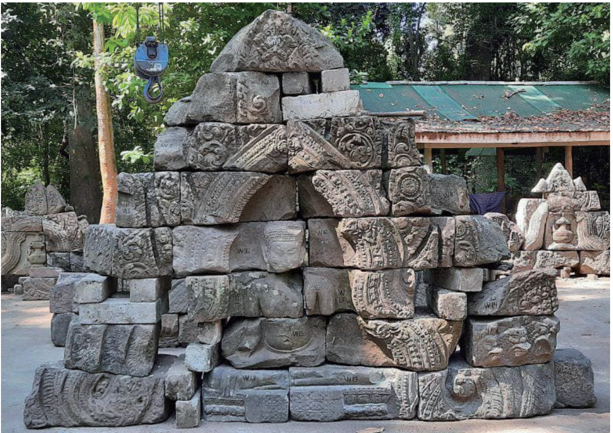
Fig. 14 Trial reassembly of the first west pediment
