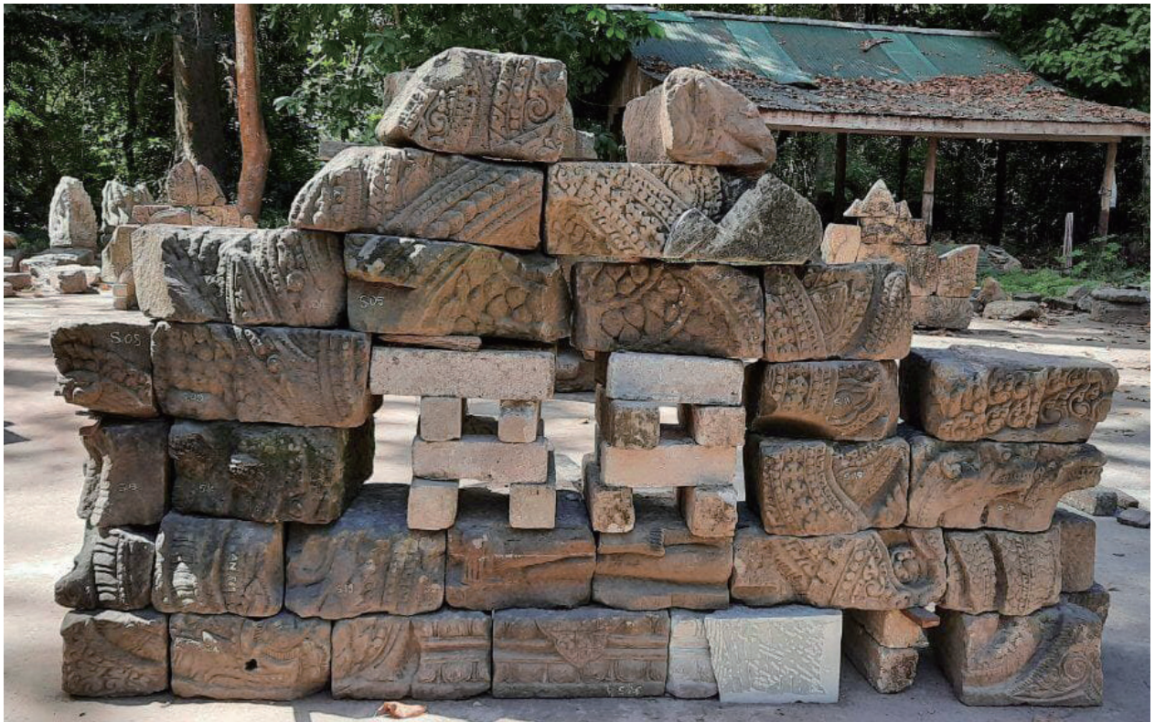
Fig. 15 Trial reassembly of the first south pediment
