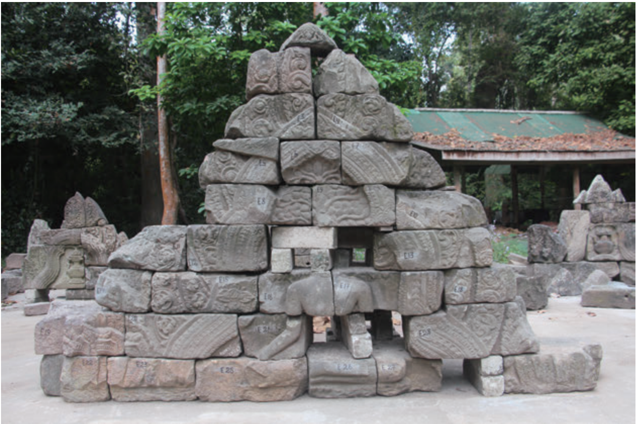
Fig. 13 Trial reassembly of the first east pediment
