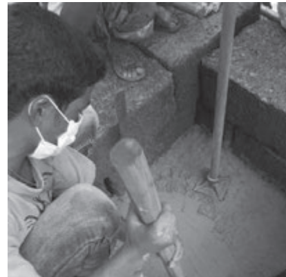
Photo 17: Compacting using an "elephant's foot" rammer
