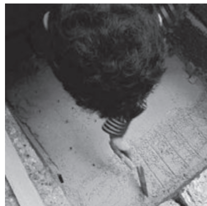
Photo 20: Delamination prevention of the compacted soil surface
