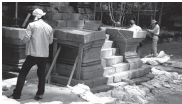
Fig. 3: Survey by the Architecture Unit
