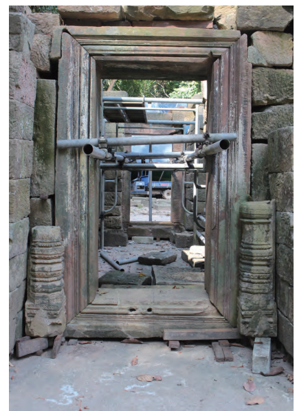
Fig.6 Eastern door frame (during reconstruction)
