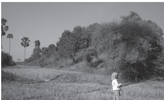
Fig.55 West earthen walls (viewed from the south-southwest)
