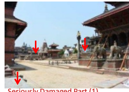
Seriously Damaged Part (1)
