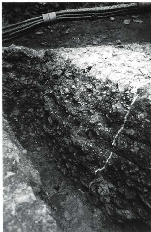
▶ 3. 2区根固め1の版築状況
