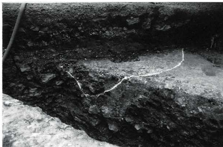
▶ 3. 2区根固め1の版築状況
