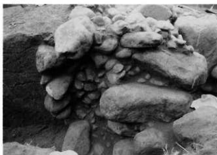
掘り方・裏込め (右側壁)
