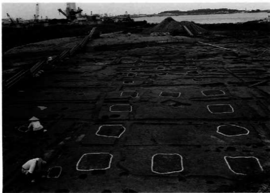
SB802検出状況
