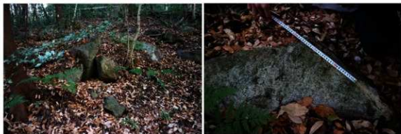
③松ノ丸東側下段帯曲輪北東側残石 左：全景、右：築石矢穴痕
