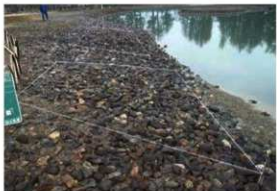
[写真 3-3-12] C区施工前
