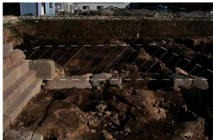
① 3240W (北側石垣台西面)
