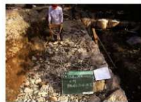
E列裏込め工
