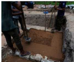
Fig. 8 Compacting the consolidated soil
