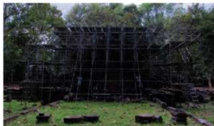
Fig. 2 View of scaffoldings (view from the east)
