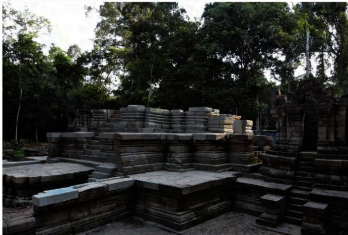
Fig. 27 View of the reassembled platform of the central sanctuary (view from the northeast)
