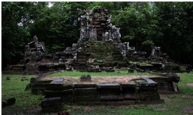
Fig. 1 Western Prasat Top before the restoration (view from the east)
