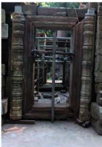
Fig.7 Western door frame (during reconstruction)
