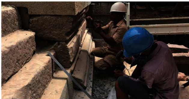
Fig. 24 Curving the new stone blocks for the central sanctuary
