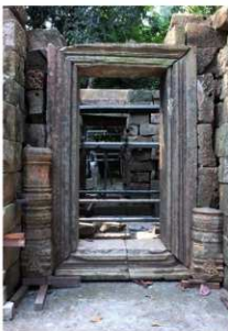
Fig.8 Northern door frame (during reconstruction)
