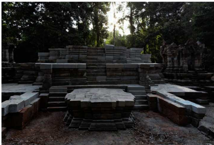
Fig. 26 View of the reassembled platform of the central sanctuary (view from the east)
