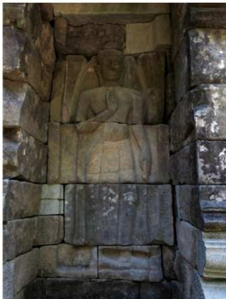
Fig. 16 Reassembled west false door of the northern sanctuary (view from the west)
