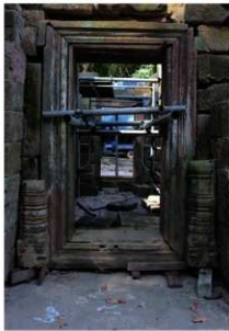
Fig.6 Eastern door frame (during reconstruction)
