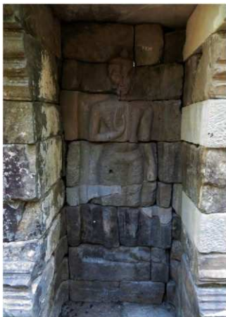
Fig. 17 Reassembled south false door of the northern sanctuary (view from the south)
