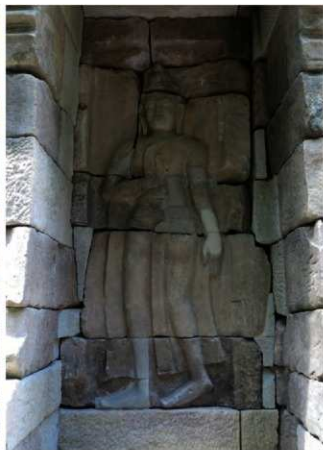
Fig. 18 Reassembled north false door of the northern sanctuary (view from the north)
