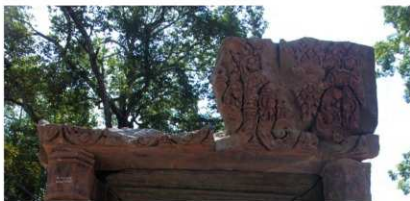
Fig.16 Northern lintel (under reconstruction)
