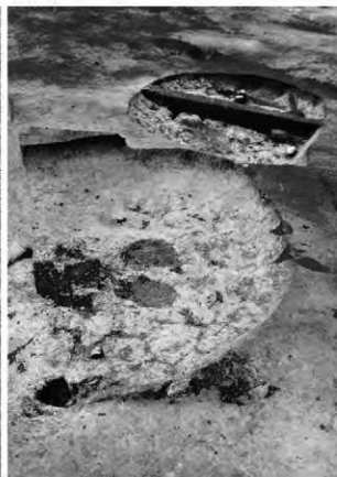
BH-7 (手前)・BH-12(奥)
