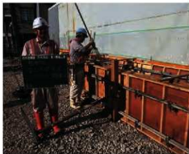
植樹枠施工状況
