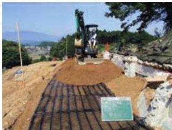
Fig.104 補強材施工状況
