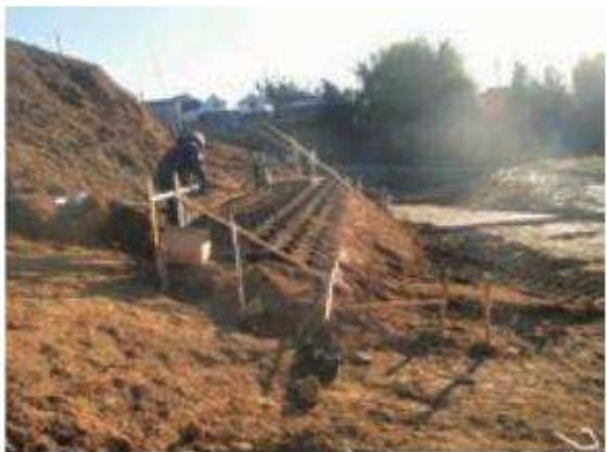
Fig.108 補強土壁施工状況（園路西斜面）①
