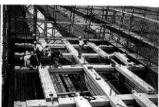
桁行台輪組立て
