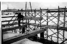
桁行台輪組立て
