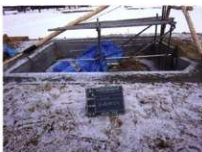
垂木基礎打設，棟組上げ
