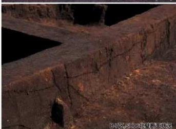
B-7区,SH06柱基断面状况
