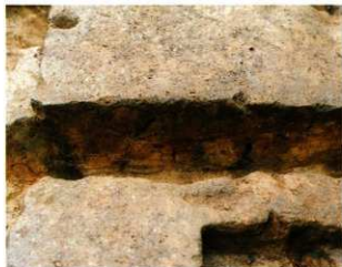
PL168 6号壑穴建物跡試掘溝H断面e-e' (分層後) Section e-e' in test trench H of pit type building No.6(lined)
