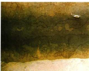
PL71 西侧扩张区西断面道路B(分層後) The section of the remain of the path B in west side section of the west extent area(lined)
