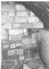
写真-139 炉下(下焚口側)
