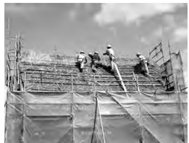
20-12 茅屋根工事①
