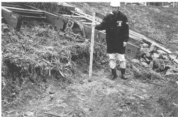
図97 鑿井工事立会調査
