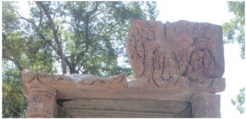
Fig.16 Northern lintel (under reconstruction)
