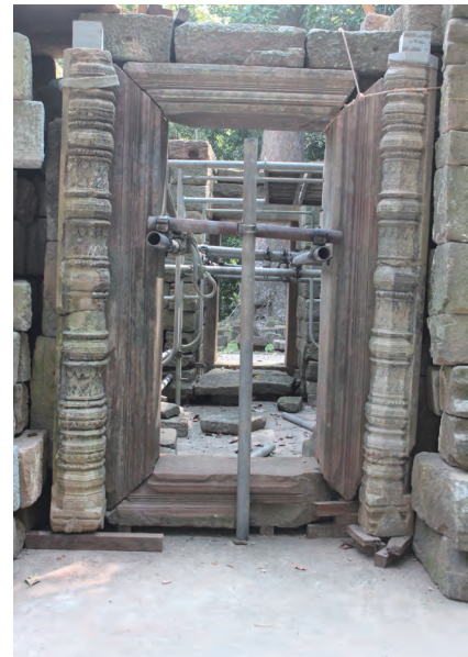
Fig.7 Western door frame (during reconstruction)
