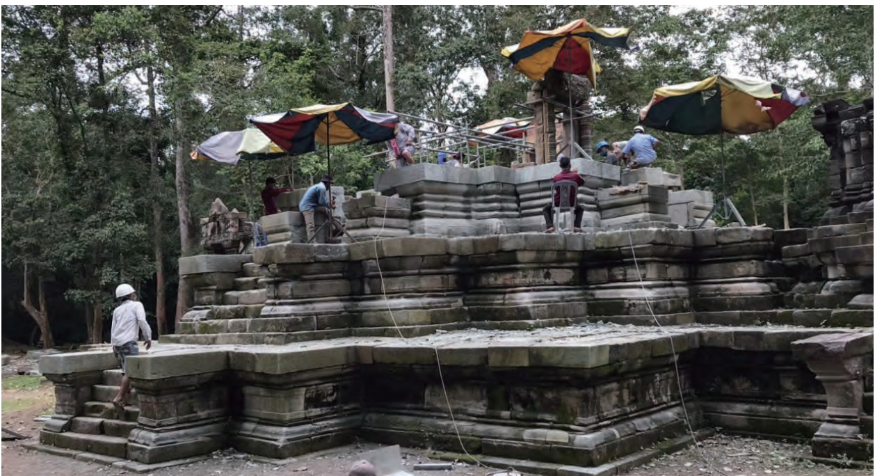
Fig. 25 View of the reassembly work of the central sanctuary
