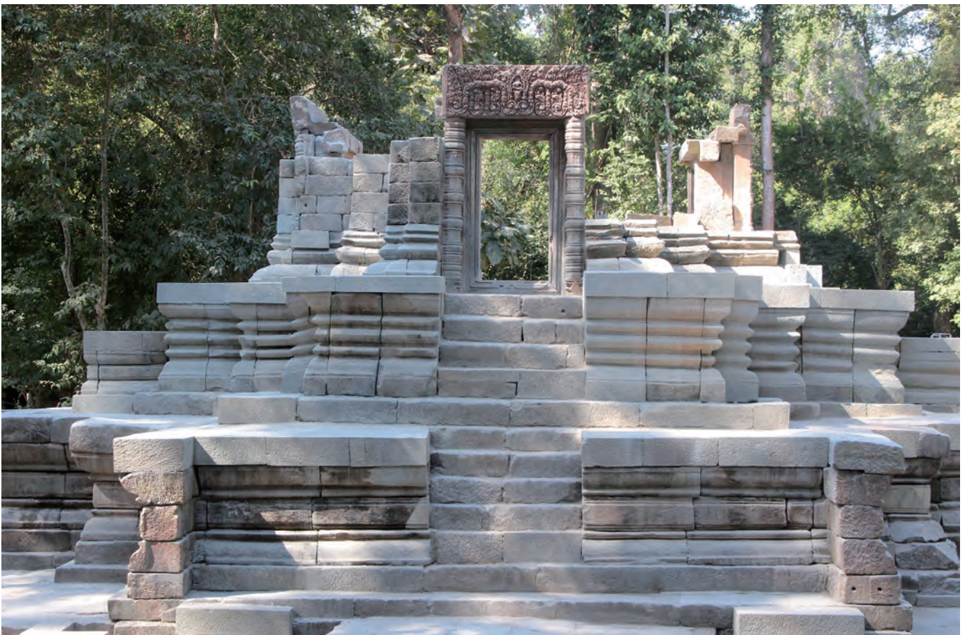
Fig. 29 View of the reassembled middle and upper platform and façade of the central sanctuary (view from the east)
