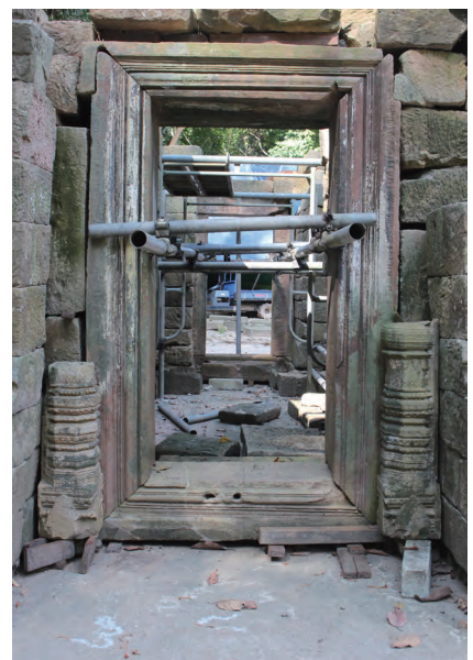
Fig.6 Eastern door frame (during reconstruction)
