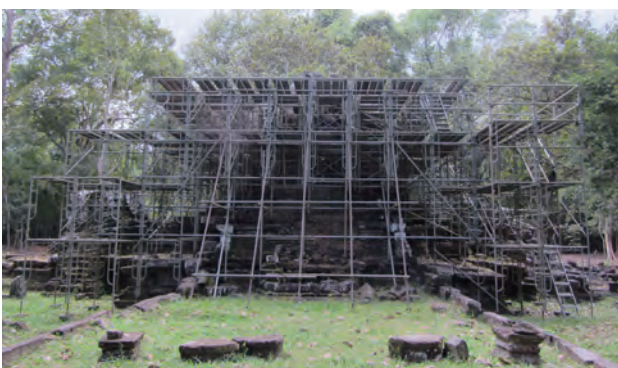
Fig. 2 View of scaffoldings (view from the east)
