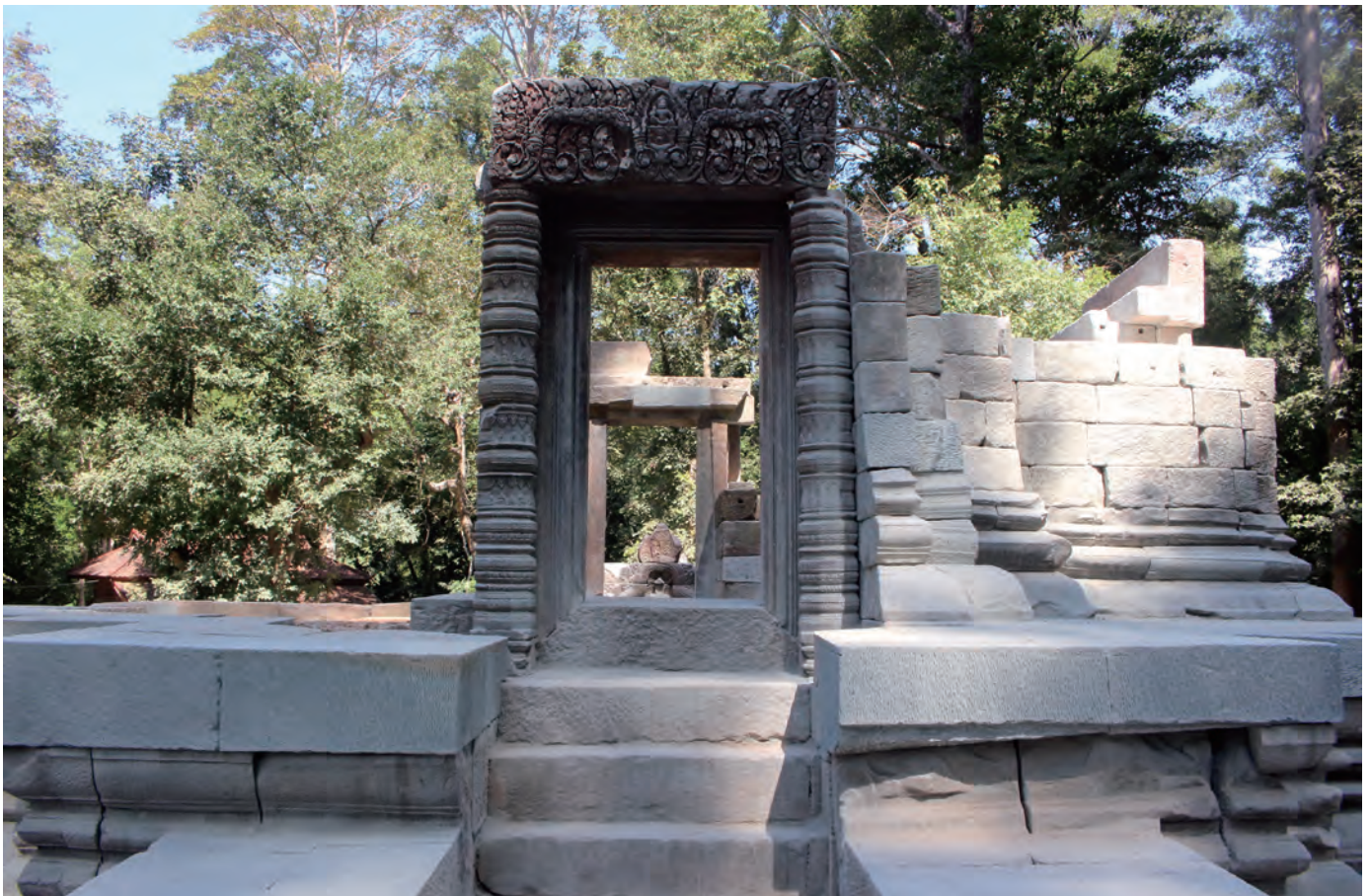
Fig. 31 View of the reassembled south façade of the central sanctuary (view from the south)
