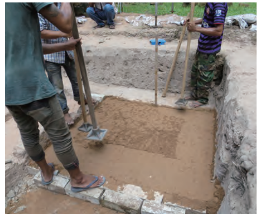
Fig. 8 Compacting the consolidated soil
