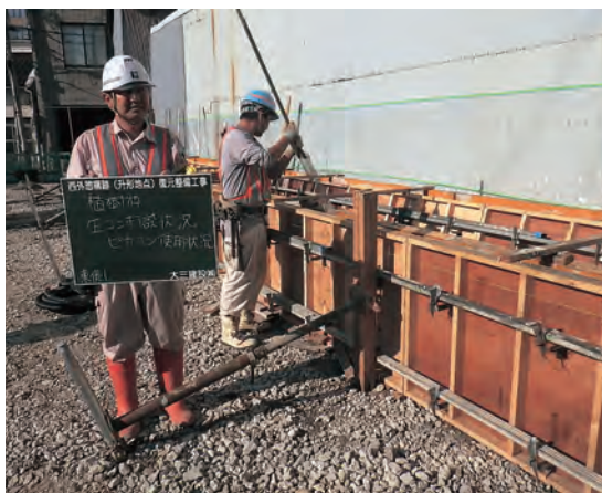
植樹枠施工状況
