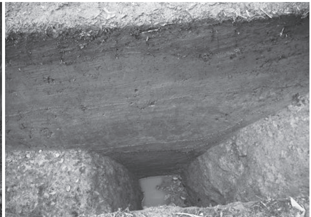
K 堀内部の南側堀
