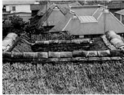
② ロの字型の屋根 (45 川副町)
