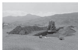
試掘坑表土の掘削
