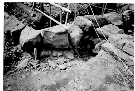
B・C面入隅部根石の飼い石と裏込めは築城時か
