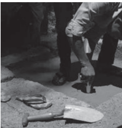
Photo 19: Compaction control using a Yamanaka hardness meter
