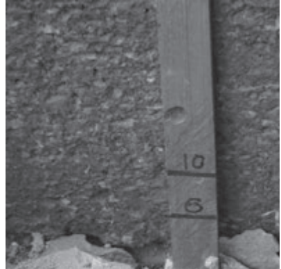
Photo 15: Soil spreading thickness and compacted thickness
