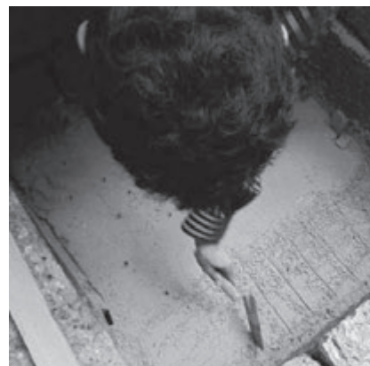
Photo 20: Delamination prevention of the compacted soil surface
