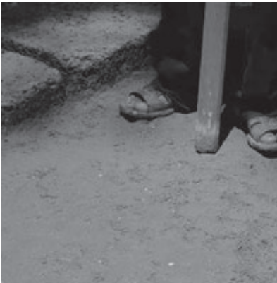
Photo 16: Leveling and compacting using a round rammer
