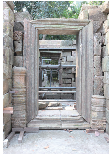
Fig.8 Northernn door frame (during reconstruction)
