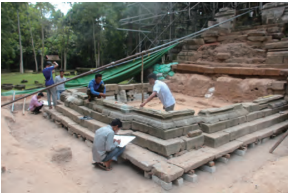
Fig. 14 Reassembly of the northern sanctuary
