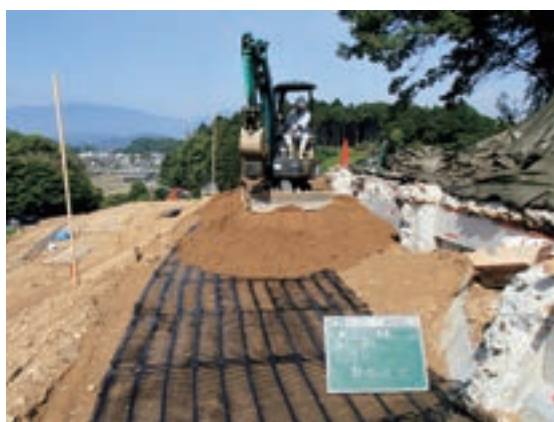
Fig.104 補強材施工状況
