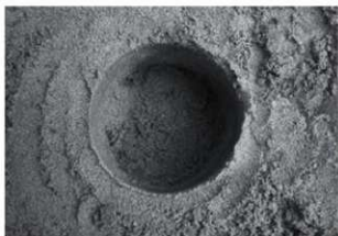
Photo 8: Erosion of the material of the lower platform
