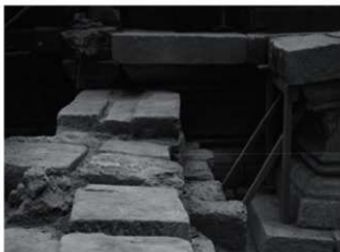
Fig. 10: Connecting area with the Central Sanctuary (view of west side)
