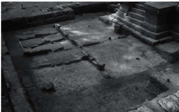
Fig. 57: Digging work and the stone lines in the foundation (viewed from the southeast)
