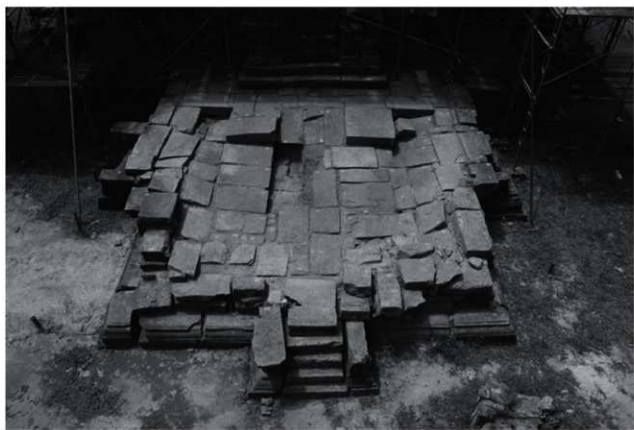
Photo 5: Subsidence of the paving stones on the surface of the lower platform
