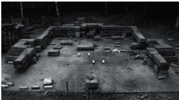
Fig. 75: Trial assembly of the lower platform (viewed from the west; June 10, 2014)
