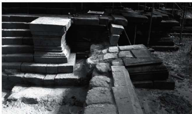
Fig. 7: Northeast corner of the lower platform
