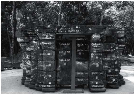
Photo 1: Temporary assembly of the main structure of the South Sanctuary
