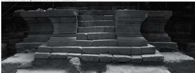
Fig. 37: South stairways of the Central Sanctuary after restoration
