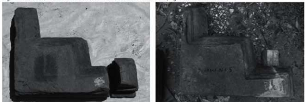
Fig. 46: Restoration of stone block SN101N15 left: before restoration; right: after restoration
