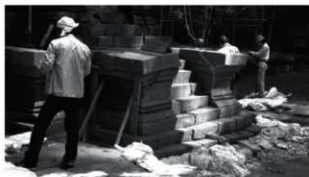
Fig. 3: Survey by the Architecture Unit
