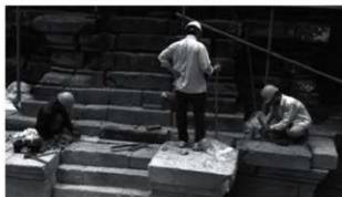
Fig. 1: Restoration of the south stairways of the Central Sanctuary
