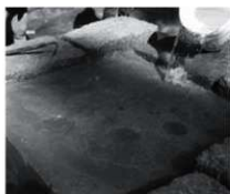
Photo 26: Water supply test after curing
