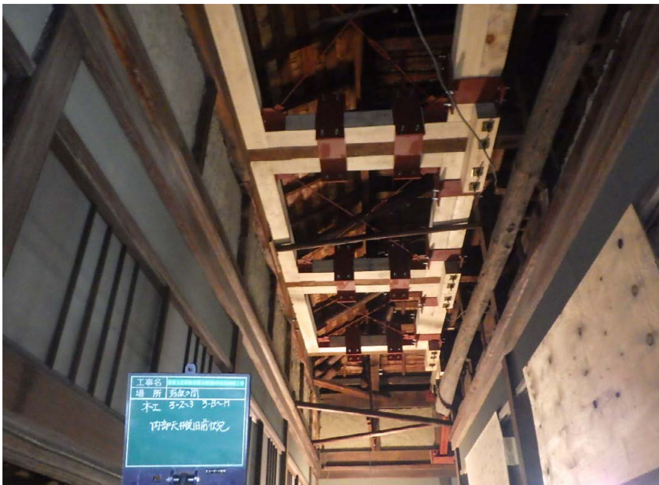
廊下側天井 補強の状況
