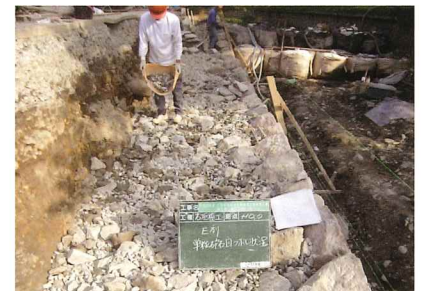
E列裏込め工
