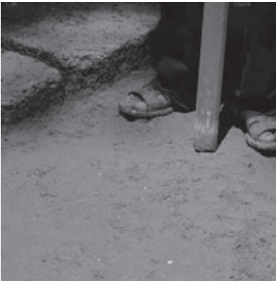
Photo 16: Leveling and compacting using a round rammer
