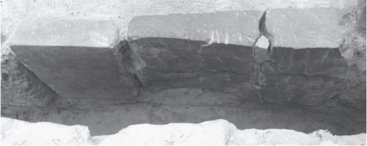
Fig. 49: Stone line in the foundation north cross-section (viewed from the west)
