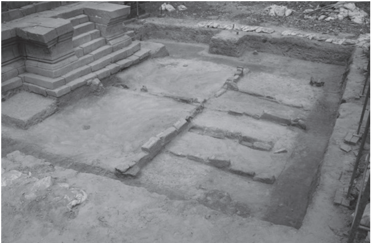
Fig. 56: Digging work and the stone lines in the foundation (viewed from the southwest)
