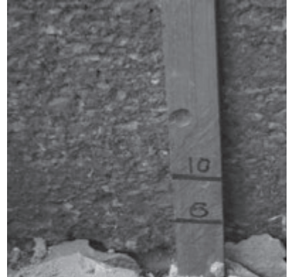
Photo 15: Soil spreading thickness and compacted thickness
