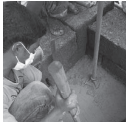
Photo 17: Compacting using an "elephant's foot" rammer
