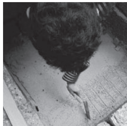
Photo 20: Delamination prevention of the compacted soil surface
