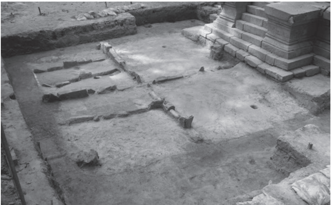
Fig. 57: Digging work and the stone lines in the foundation (viewed from the southeast)
