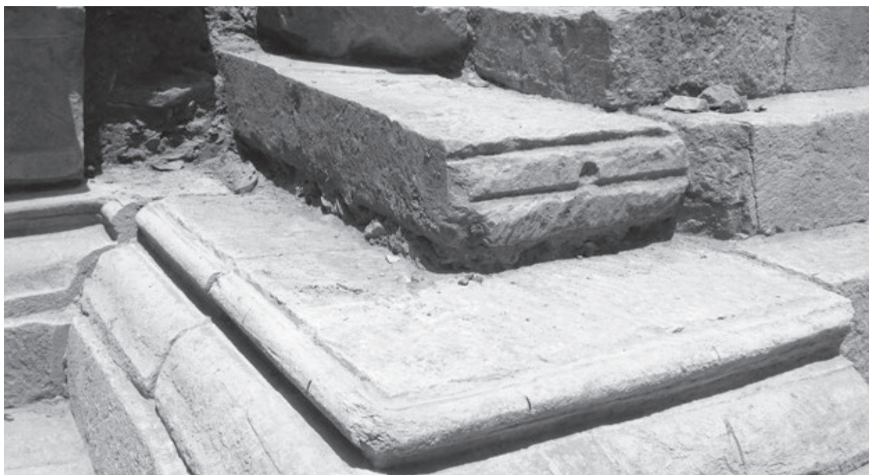
Fig. 43: South stairways of the Central Sanctuary diverted stone blocks on the inner side of the west sleeve area
